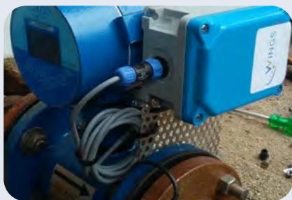
WINGS Nb-IoT based device for enabling smart water management, consumption monitoring/predictions and fault management
